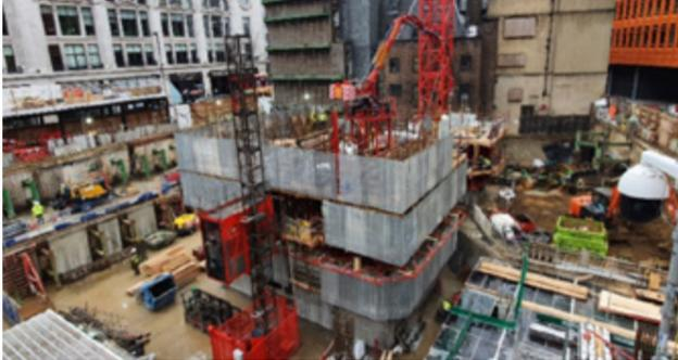
Slipform reinforced lift & stair core construction
