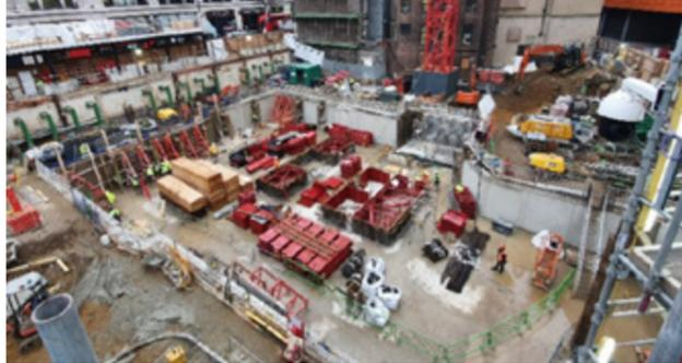
Completion of basement 2 structure and Slipform mobilisation
